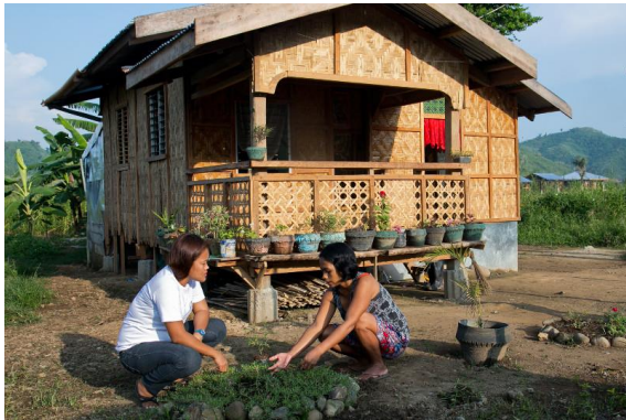
Shelters designed by CRS engineers are adaptable to people's needs as their lives change and improve, with the ability to add rooms and floors. Photo by Jen Hardy/CRS
